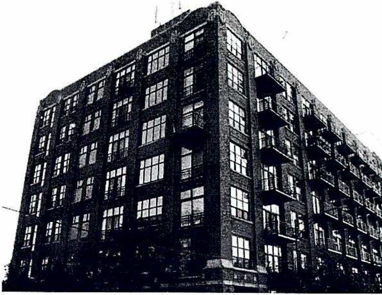
Figure 4. Southwest corner of building
