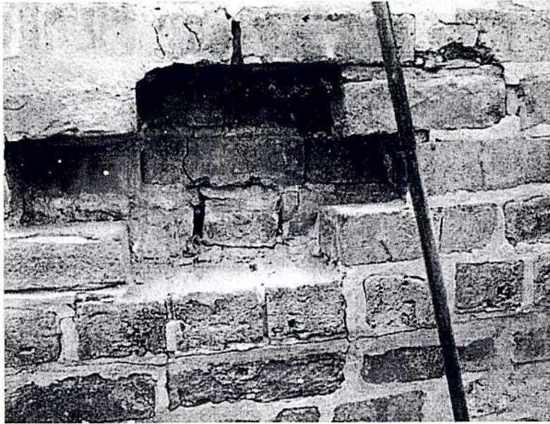
Figure 13. Inspection opening at parapet along north elevation.
